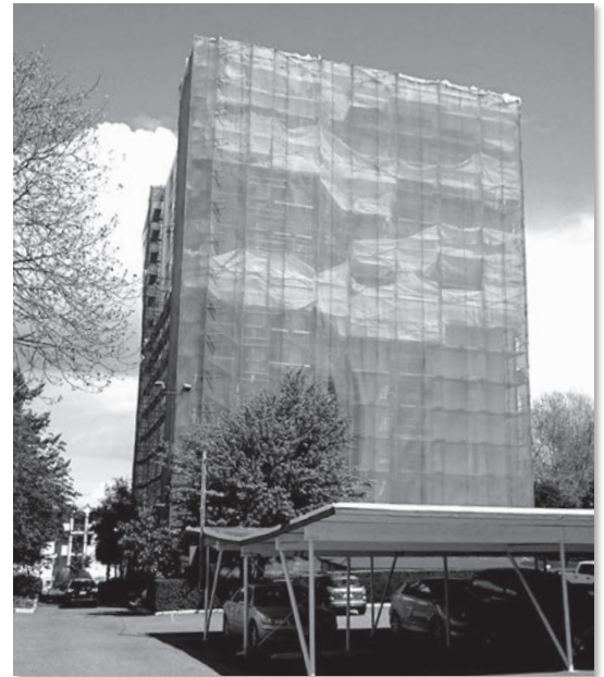
The Starlight building on Michigan Avenue is covered for renovations.
