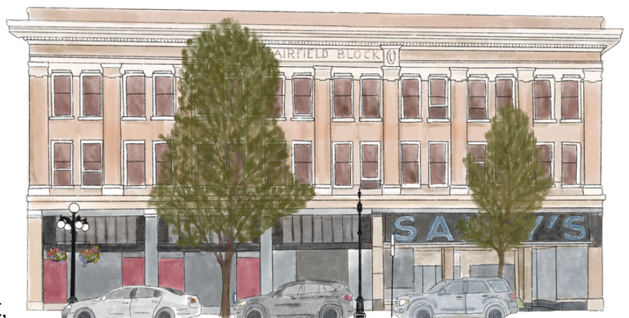
PICTURED: THE FAIRFIELD HOTEL ON DOUGLAS STREET, ONCE A VICTORIA SRO THAT CLOSED IN 2019, RESULTING IN THE DISPLACEMENT OF DOZENS OF TENANTS.
